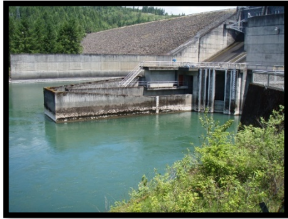
Above Foster Dam
